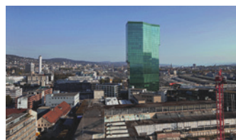
Prime Tower Zurich, Switzerland
