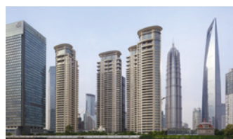
Tomson Riviera Apartment Towers Shanghai, China
