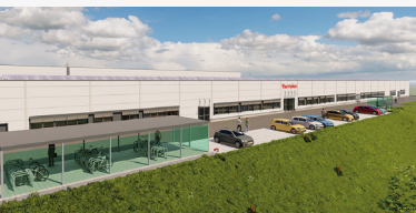
Production and Warehouse (11.000 m 2 ) in Bischoffen
