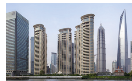
TOMSON RIVIERA APARTMENT TOWERS SHANGHAI, CHINA
