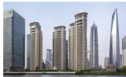
TOMSON RIVIERA APARTMENT TOWERS SHANGHAI, CHINA
